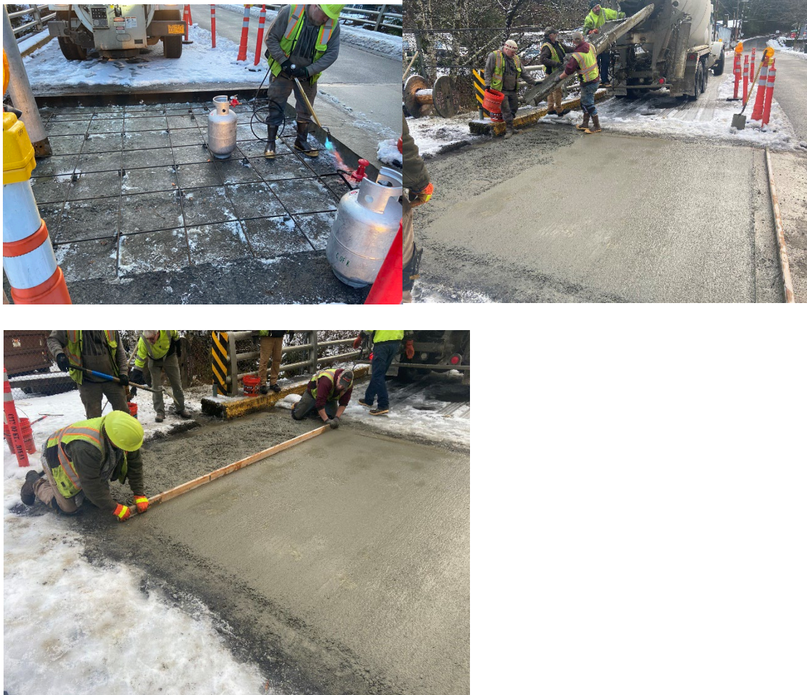
Concrete Pour at Fair Street Bridge Approach
